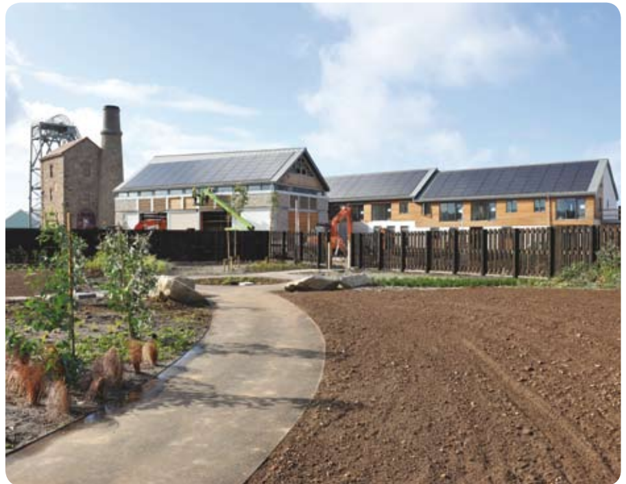
New PV panels on the roofs at Heartlands
