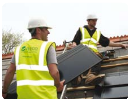
Co-op members installing a PV system
