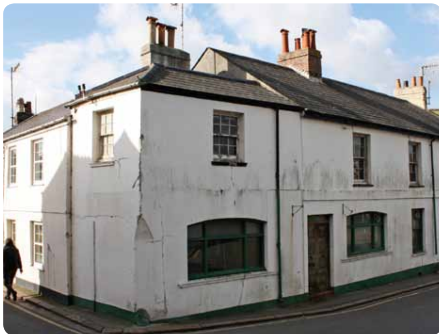
The building before renovation started
